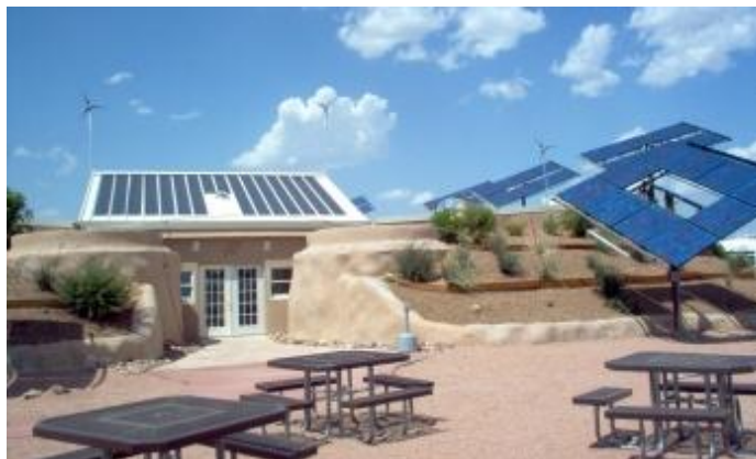
Solar panels on Award Winning Environmental Office, AZ ARNG.
