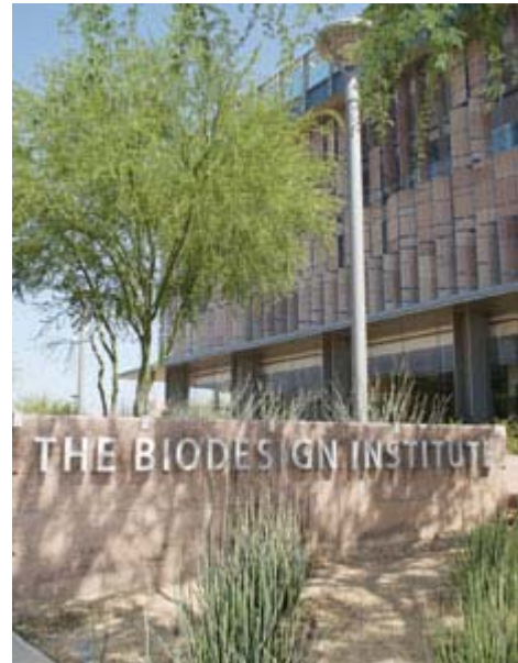
ON THE ROOFTOP: University officials announced plans June 10 for a series of rooftop solar panels to be installed on top of the Biodesign Institute.
