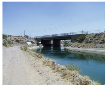
Figure 3: View SE from north side of canal, looking at the Shea bridge (Shea runs E/W). This area is considered stable (it has not subsided or has subsided only slightly). The cement liner starts halfway between the road and the water surface. "Freeboard" is this exposed part. At this location, there is ~4ft of freeboard. Photograph by J Ramón Arrowsmith.
