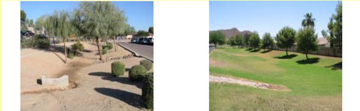
Figure 1: Examples of xeriscaped (left) and grassy (right) stormwater retention basins. Xeriscaped basins frequently have drip-irrigated vegetation on the upslope. Grassy basins must be irrigated frequently to maintain greenness.
