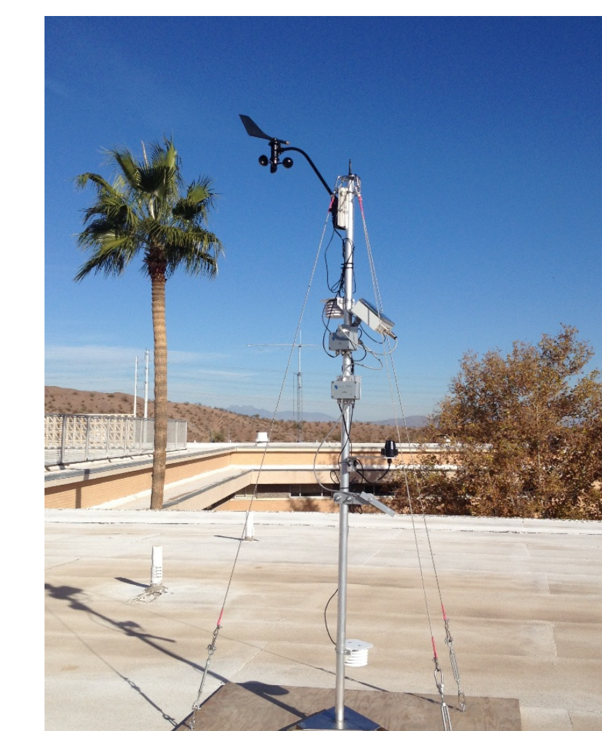
ASU's CSB roof (white roof)
